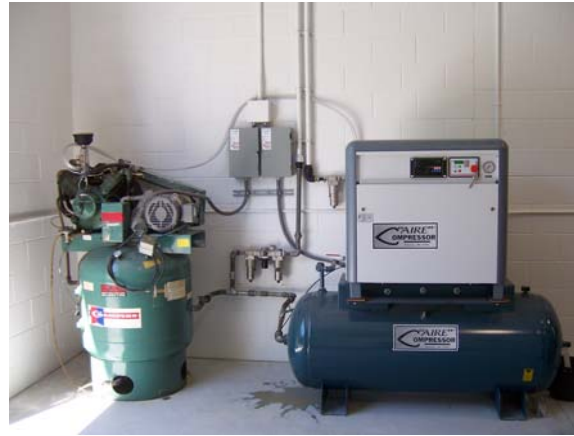
The compressor retrofit
